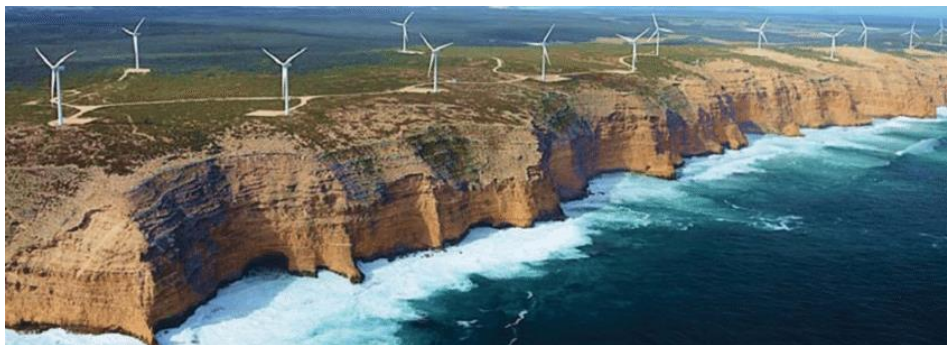
South Australia is Australia's leading wind power-producing state
