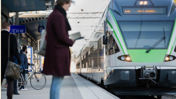
Finland's electricity-driven railway network covers all major cities in the country, reducing carbon emissions
