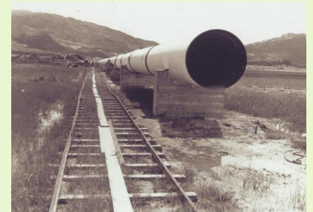
In order to hold the water transported from Shenzhen Reservoir, Hong Kong laid large water pipes in 1960.
