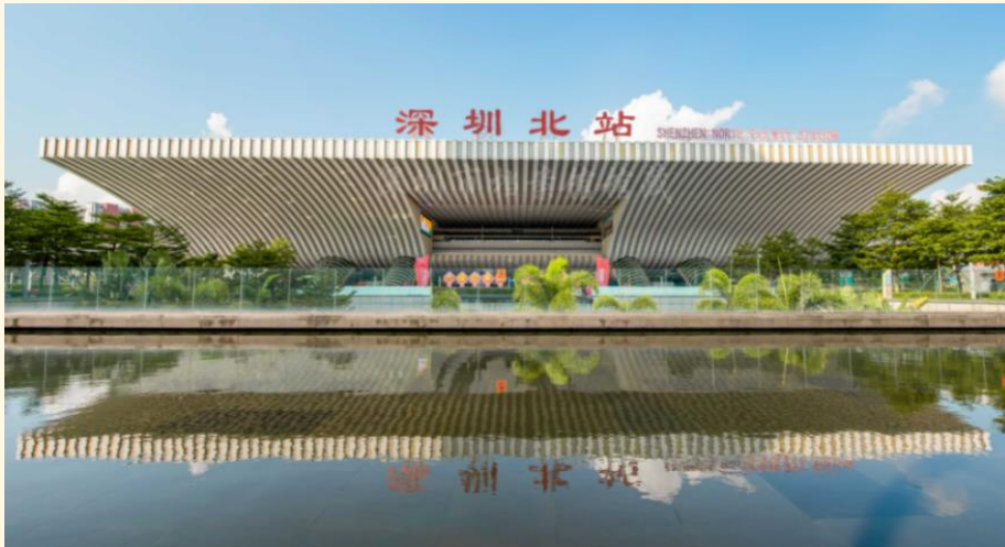
Shenzhen North Railway Station
